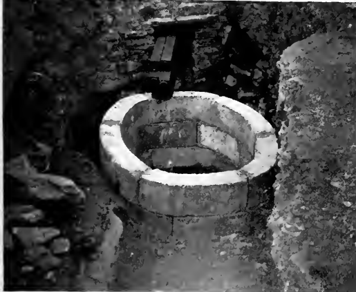
FIG. 2.—GENERAL VIEW OF BLOCK MANHOLE.
